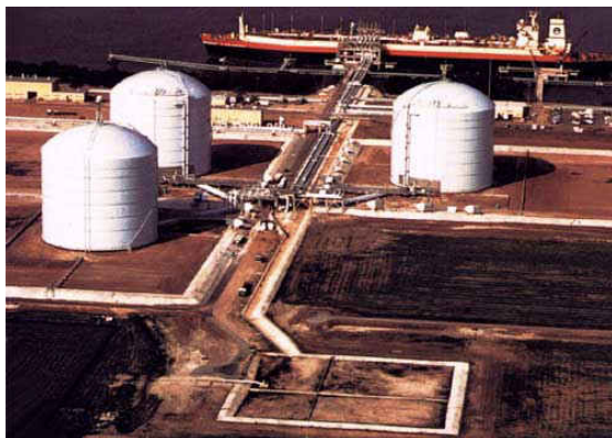
Elba Island Import Terminal, Georgia Photo Courtesy of CH-IV International, http://ch-iv.com
